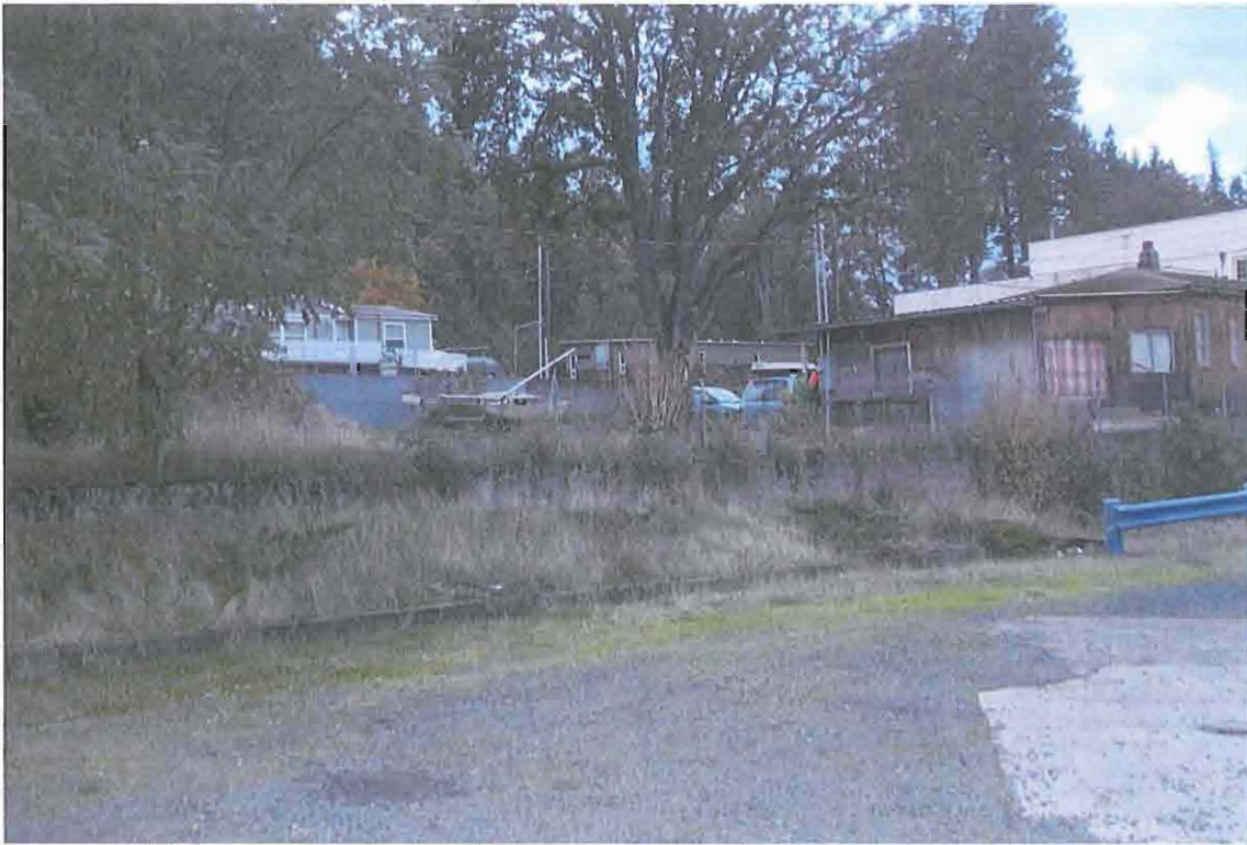
Former Mosier Motel Looking South From Mosier Gas Site
