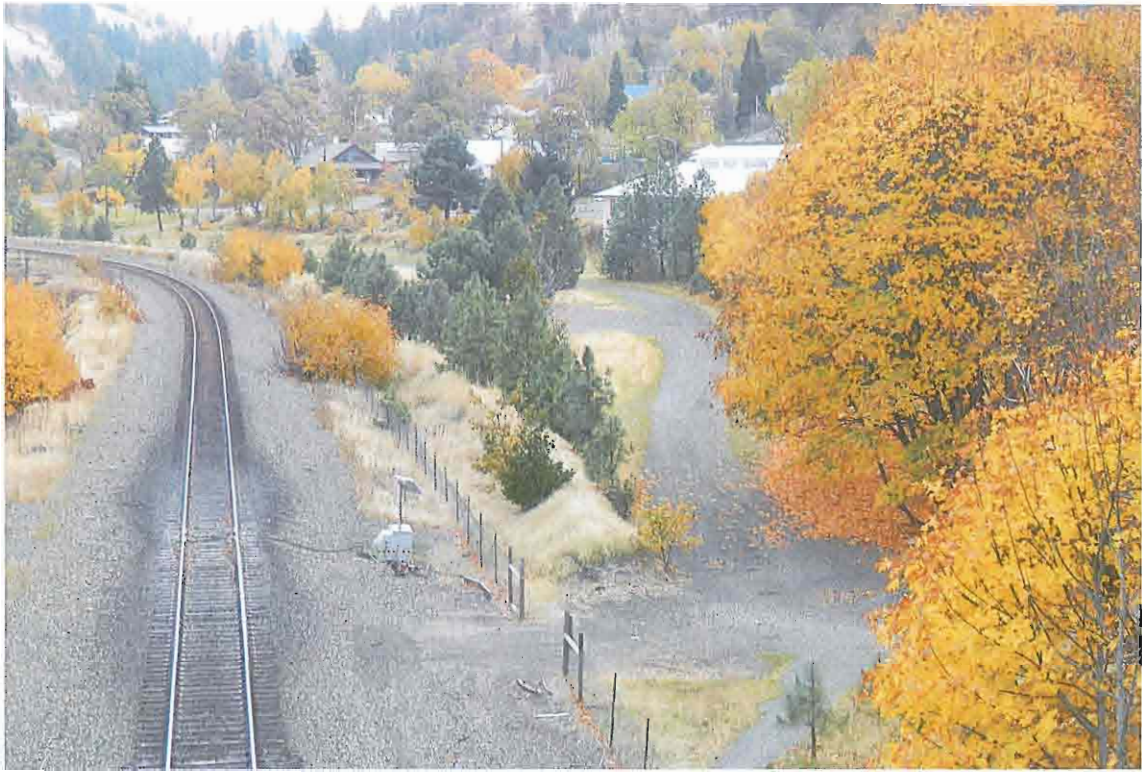
Overview of UPRR Site Looking East-Southeast from Overpass
