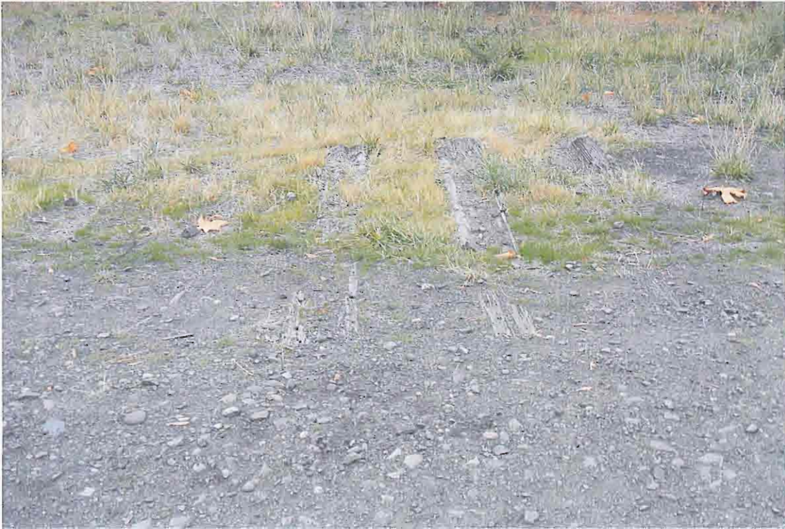
Railroad Ties Remaining in Ground in Central Portion of UPRR Site
