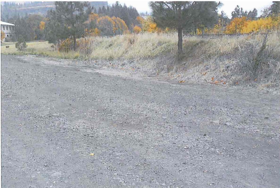
Central Portion of UPRR Site Looking NE at Tire/Soil Berm
