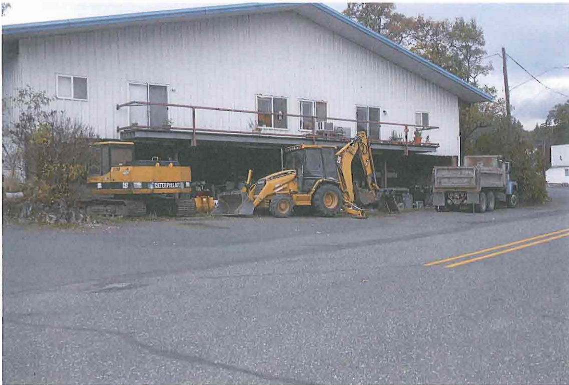
Kennedy Excavating Site
