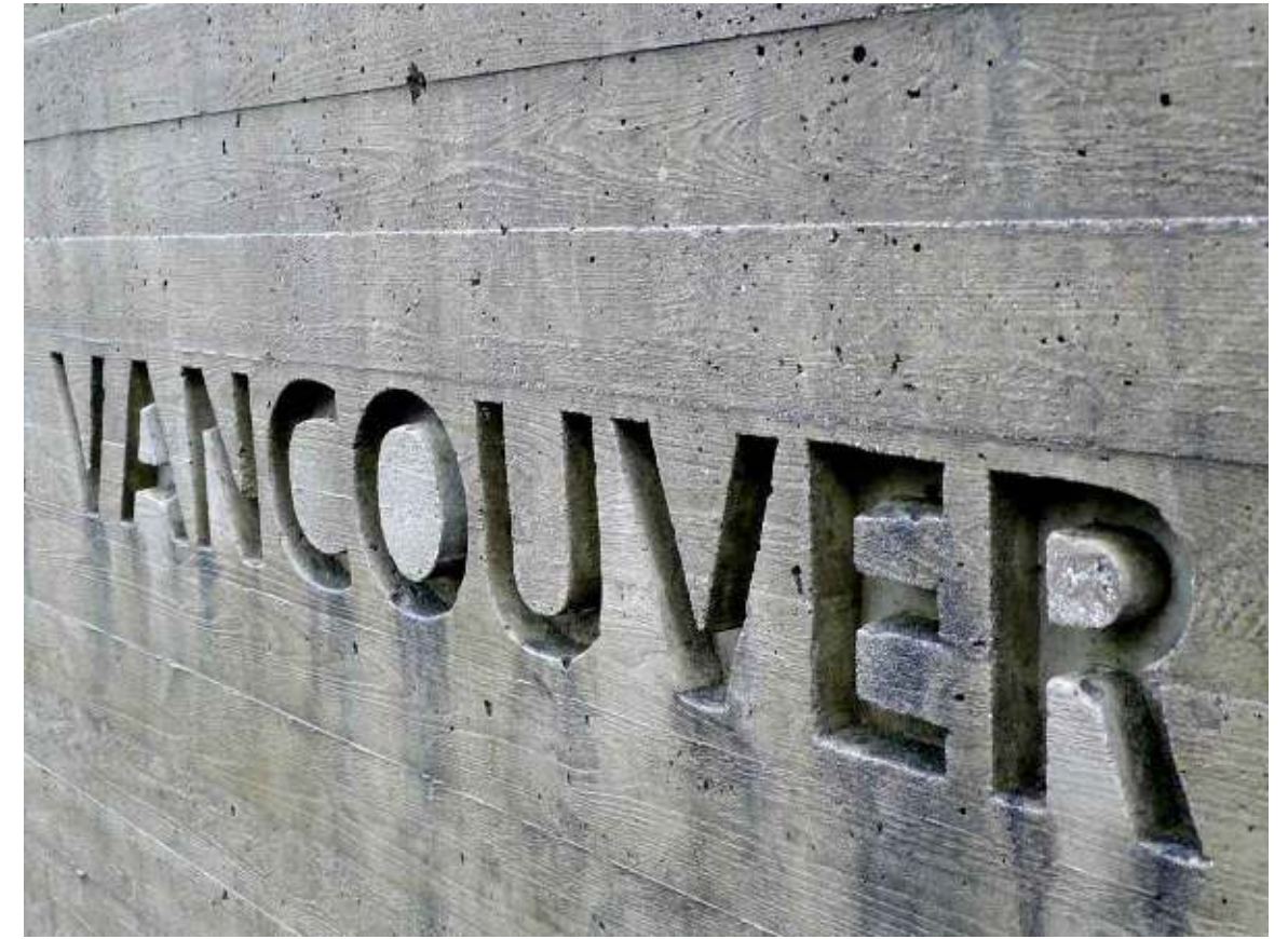
BOARD FORMED CONCRETE
